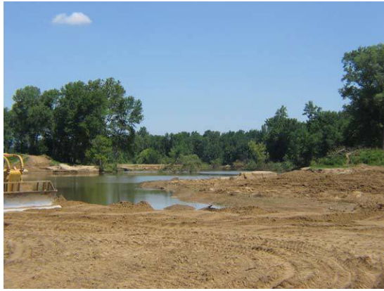
Fig. 3 Crater lake extending through 100-m levee breach.
